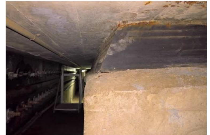
4.1-3 Elastomeric bearing at the northern portal building.
